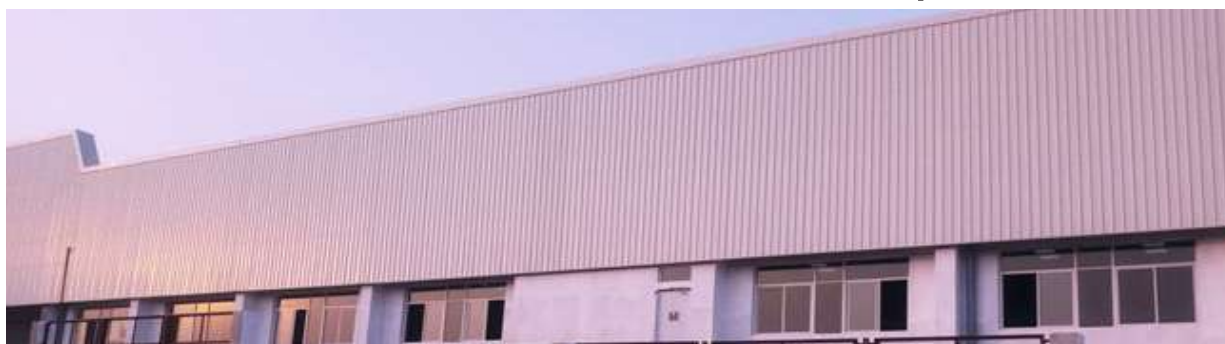
A.M. Enterprises -Chakan,Contractor-Unity Construction Pvt.Ltd.Area-5000 Sqm
