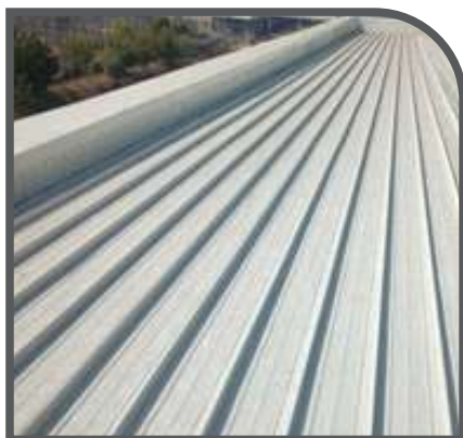
Standing Seam Metal Roof
